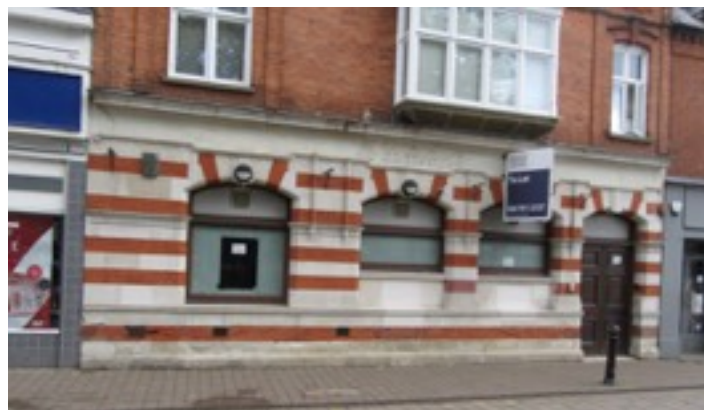
Former NatWest bank premises looking forlorn
