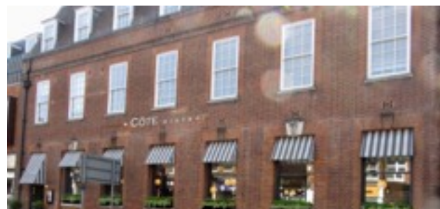
Commended: Conversion of former Post Office
