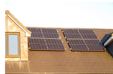
Solar roof panels
