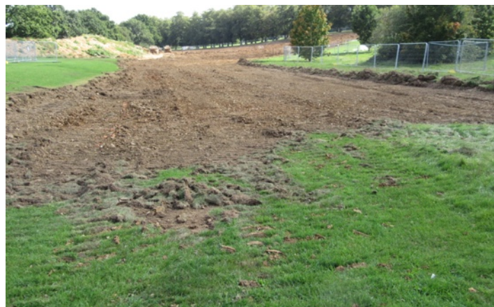
Above. Bulldozer at work on the topsoil 'mountain', with the separate subsoil 'mountain ridge', as well as the new Leisure Centre, in the background. Below: The area of the park having its topsoil removed – for later reinstatement – extends to 3.2 acres.
