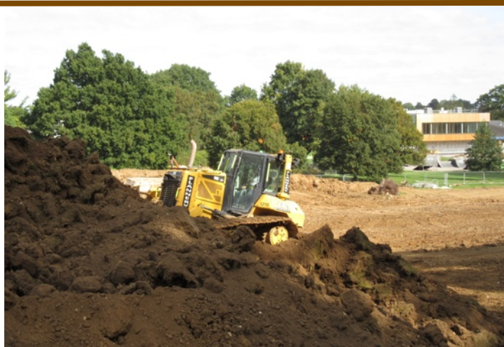
Above. Bulldozer at work on the topsoil 'mountain', with the separate subsoil 'mountain ridge', as well as the new Leisure Centre, in the background. Below: The area of the park having its topsoil removed – for later reinstatement – extends to 3.2 acres.
